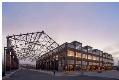
Building 12 © Bruce Damonte
